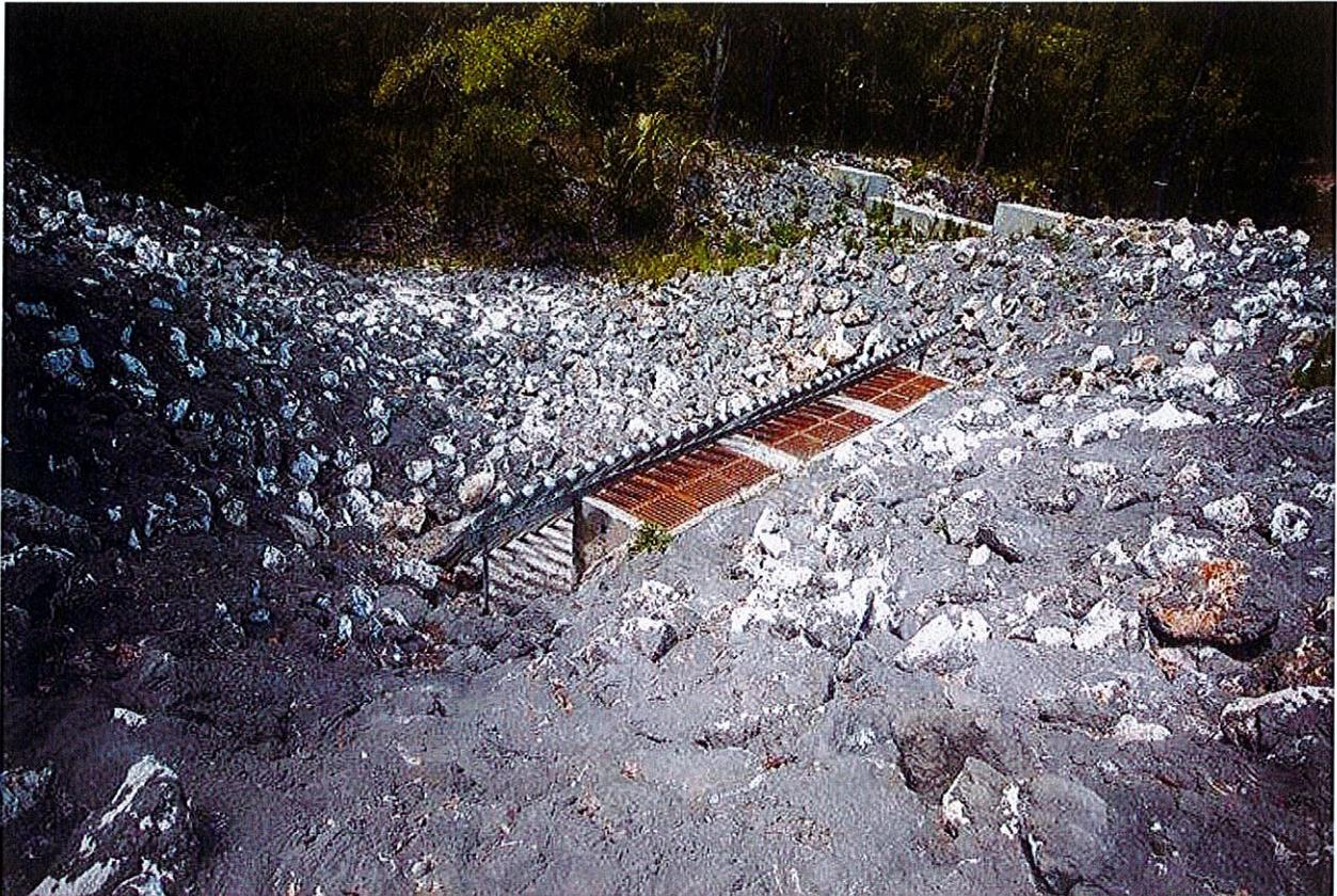
*A grate system helps to filter large items from storm water before it reaches the filtration system in the Peck Sink Preserve. OCTAVIO JONES | Times*
